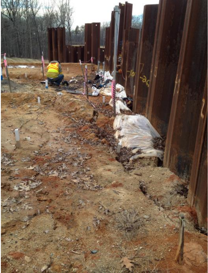
after 6.7 m excavation
