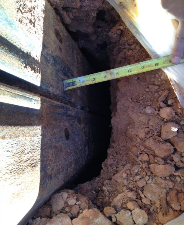
after 6.1 m excavation
